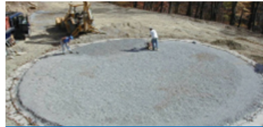
Ring Wall and Compaction
