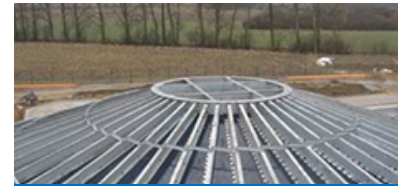
Assemble and Complete ESR Structure/Panels
