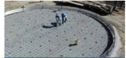
Set Slab Reinforcing Steel
