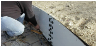
Install Foundation Seals
