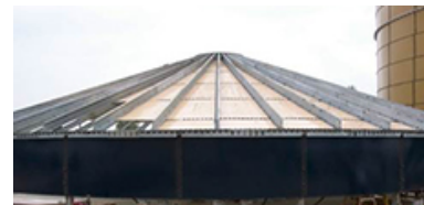
Jack and Raise Tank to Install Panel Rings
